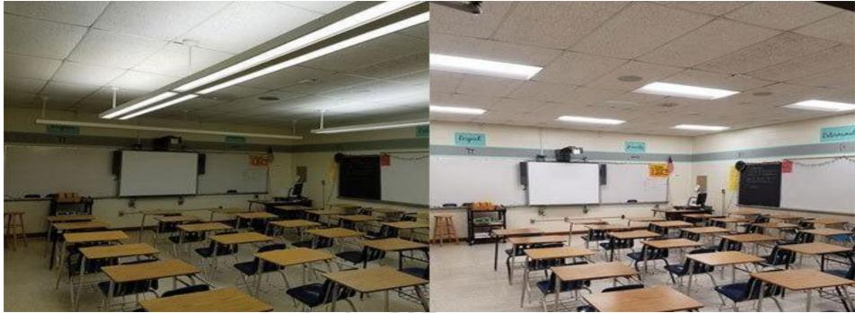
The facility was retrofitted with over 3000 LED lighting fixtures / blubs. The fixtures were available in a warm or neutral color temperature with a variety of snap-in reflector options, the LED fixture is designed to easily retrofit into new or existing fixtures. With the LED downlight's decreased energy consumption and reduced maintenance cycles, the facility is expected to recoup its costs in 6 months. The overall warranty was seven plus years or more depending on the product.
